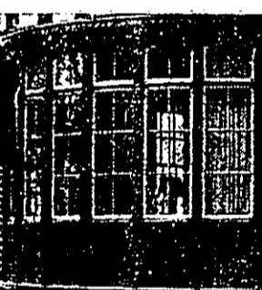
A radial bay of casement windows so popular today.
