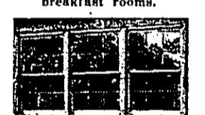
A multiple bank of double hung windows at the end of the living room.
