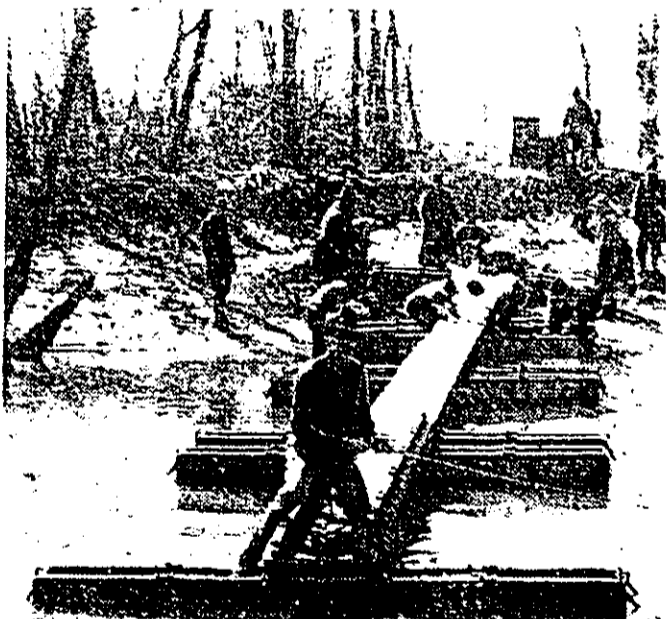
ENGINEERS BRUSH UP —Units of 121st Engineers construct 72-foot pontoon bridge across Patuxent river at Fort Meade, Md., as part of their training under U. S. defense program.
