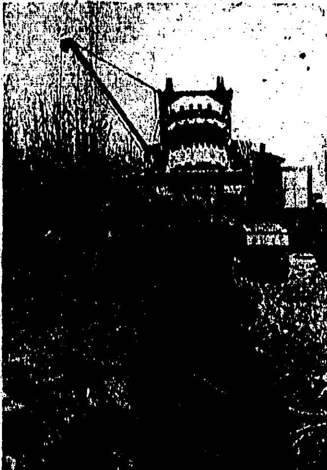
DIGGING THE "BIG DITCH" —A giant ditch-digger plows through Pennsylvania at a fast clip, taking every thing in stride as it lays an oil pipe line to Northern cities from Texas oil fields.
