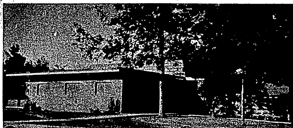
MEDICAL AND DENTAL CLINIC—The newly constructed Medical and Dental Clinic into which Drs. Robert E. Swearingen and Curtis N. Garner moved this week is pictured above. The building is located at the corner of Kelley Boulevard and Dogwood street just north of Tyler County Hospital. Dr. James Malcolm Radford, a dentist, will become associated with the clinic Monday. Open house for the general public will be held Sunday from 3 to 5 p. m.
