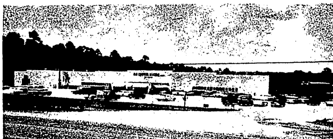
PHOTOS AT LEFT show Air Control Window Corporation's present plant at top and site of the new addition, below. Work has started on clearing this location.
