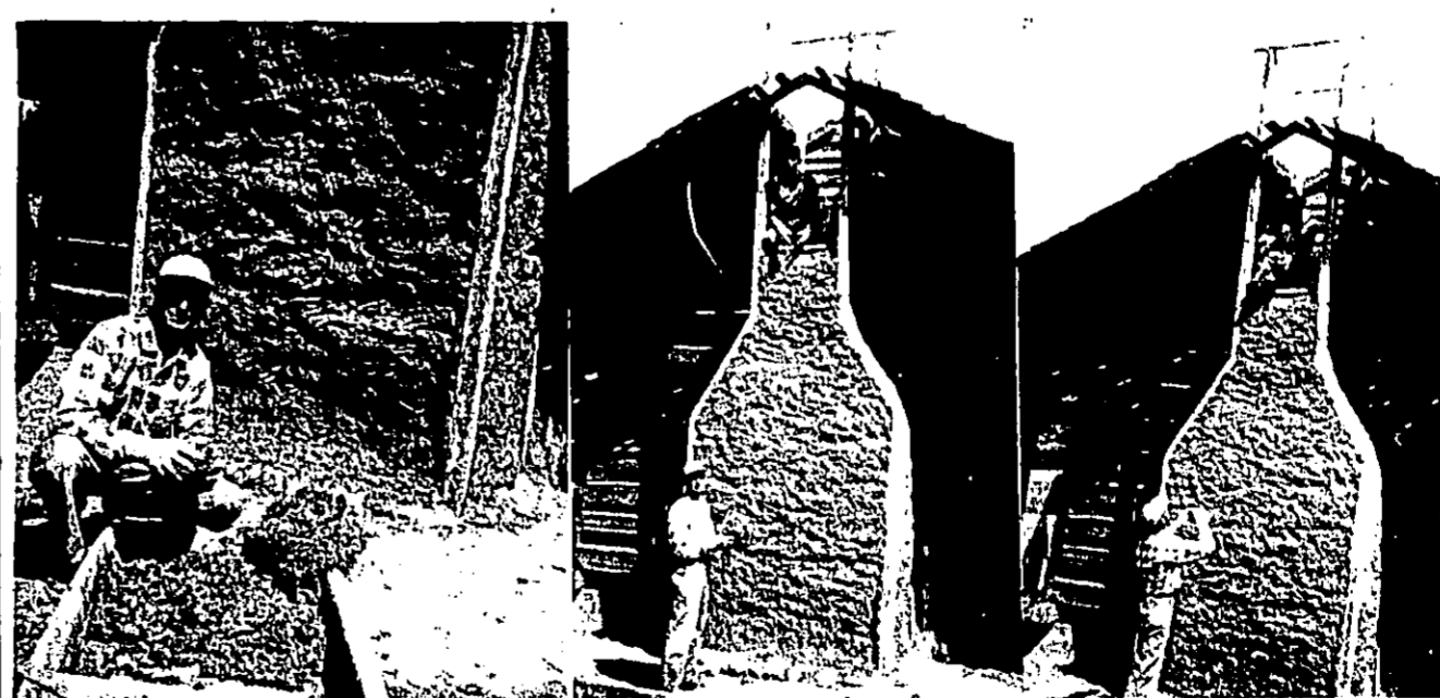
HOW TO MAKE A MUD-CAT CHIMNEY—Noah Platt and Herman Brandin demonstrate the finer points of building a "mud-cat" chimney for the Press photographer at the Tolar Kitchen at Heritage Gardens.
