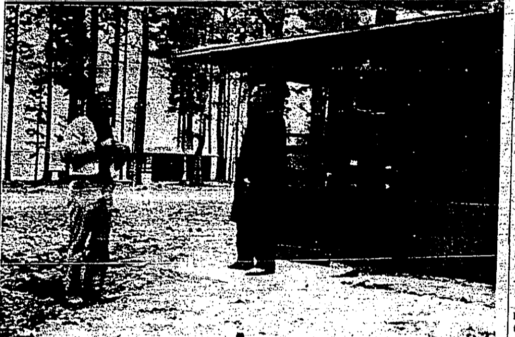
WATER TOWERS, picnic tables, and shelters are just part of the many attractions at Dam B State park now under construction. At top, workmen cling to girders of what will be a 102-foot high steel tower supporting a 20,000 gallon cypress water tank—one of two in the system. Center, inmates from the Texas Department of Corrections smooth rough edges of one of 240 concrete picnic tables in the park. Bottom, Joe Adair left, construction superintendent at the park and Parks Department official from Austin, stand before one of the 12 by 16 foot screened shelters.
