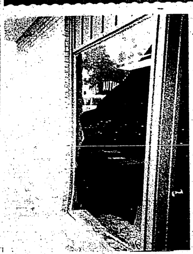
Last week an auto drove into the parking place at Community Inn in front of the Housing Authority of Woodville, the brakes failed, and the auto went through the plate glass window. Notice the curve in the brick wall at lower left which was caused by the car's bumper. J.F. Stanley, of the office, was in the office but luckily was not hit by flying glass.
