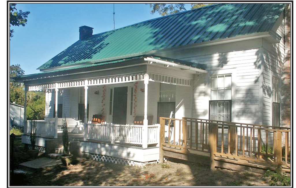
The W.T. Colmesneil House after renovation.
