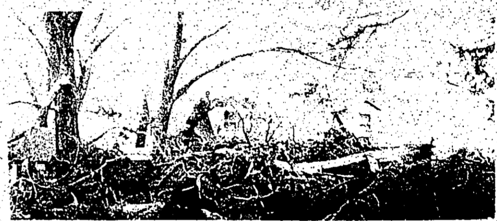
The yard at J. Wood Fain residence following storm.
