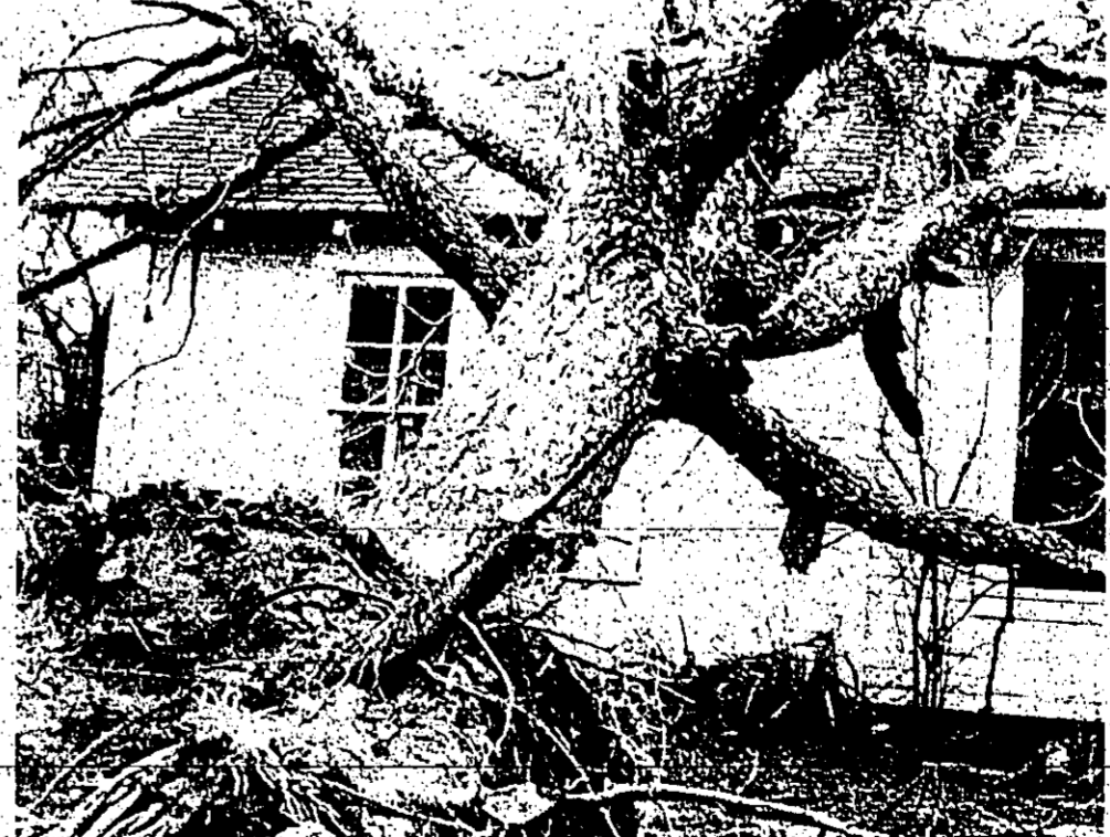
One of three trees blown down at home of Mrs. Tom Cole lands on house.
