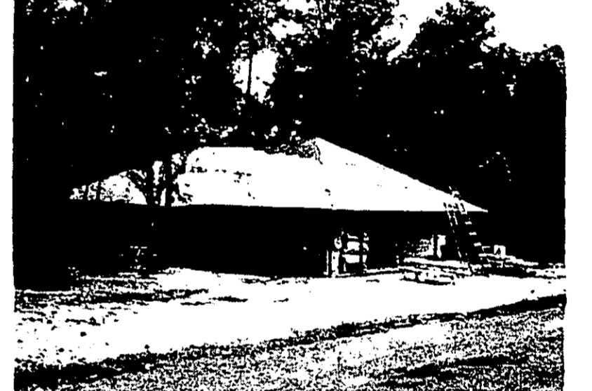
Steady progress is being made on the new office and recreation center at Big Thicket Lake Estates.
