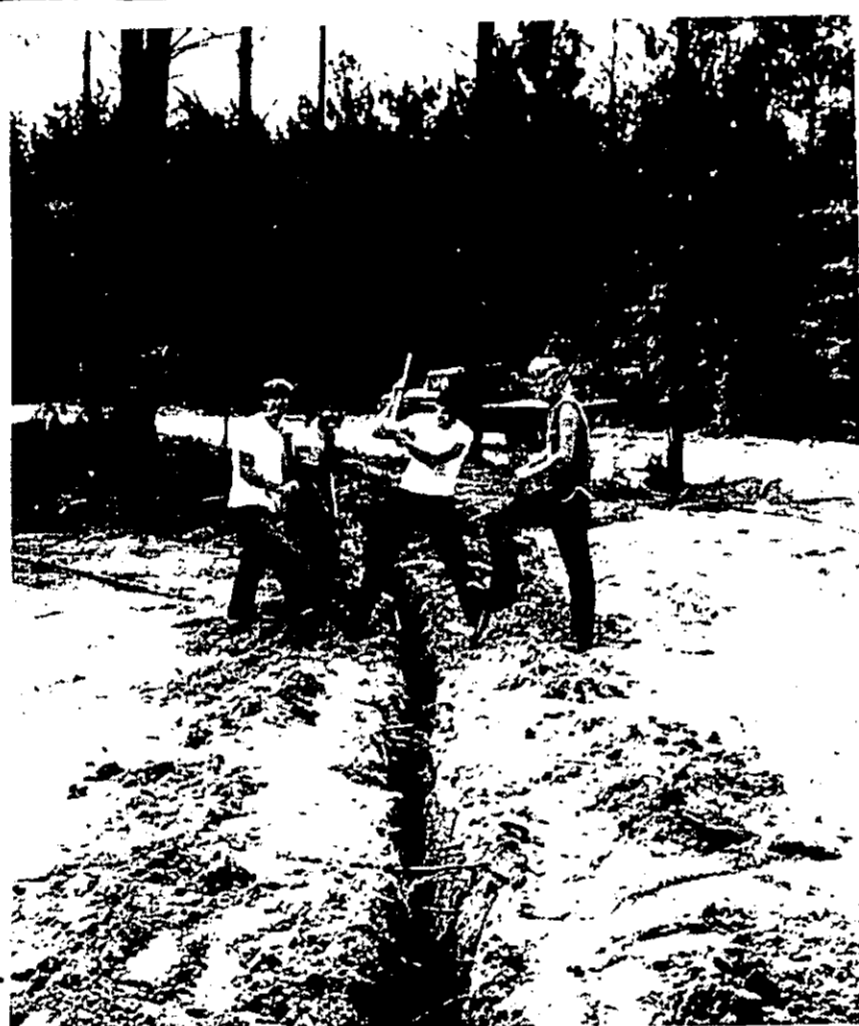
Neil Collier, Cornelius Mangum, Job Wiggins and Rex Minter, the regular working crew at Wiggins Village, putting in water lines.
