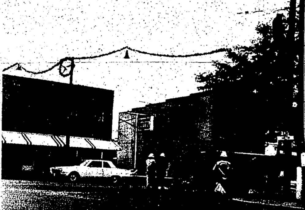
Gulf States crewmen are putting up Christmas lighting in the downtown area this week, including several new strings of lights purchased this year to add to those which have been strung in previous years. They hope to have the job done by the time you read this. The photographer did not get the name of the man on the pole (and it was 44 degrees on the ground).
