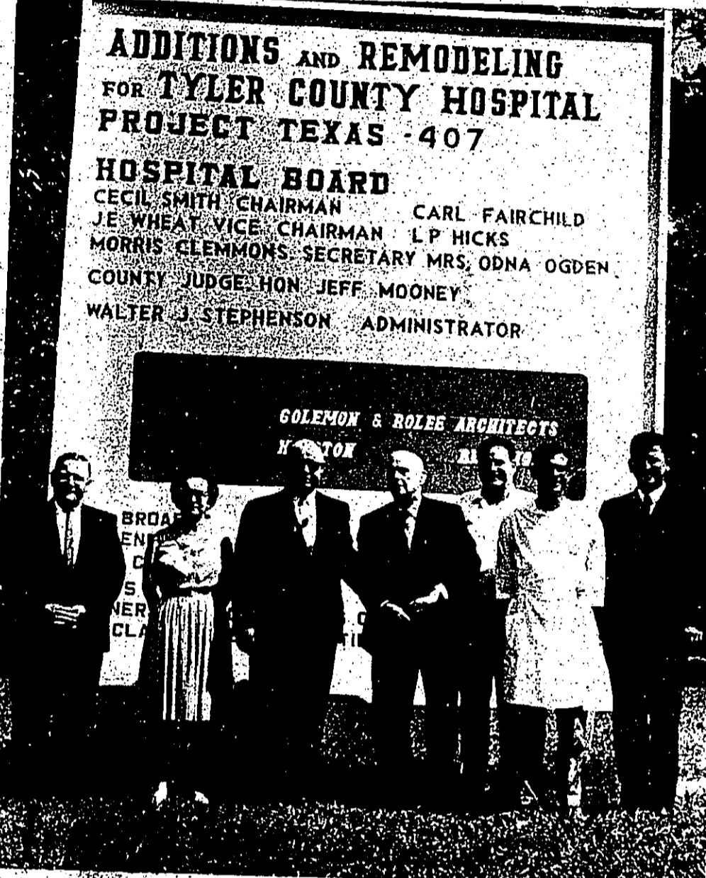
Members of the Tyler County Hospital Board are shown Monday posing before the sign designating construction which has started on enlarging and improving the facility. From left are: L. P. Hicks, Mrs. Oona Ogden, Carl Fairchild, Cecil Smith, board chairman; Morris Clemmons, Jr., secretary; Clay Miller, technician, and Jerry Stephenson, hospital administrator. Not Present were J. E. Wheat vice chairman of the board, and County Judge Jeff R. Money. (See story)
