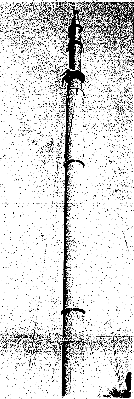
Towering over 100 feet into the air and looking for the world like a rocket ready to blast off is this center post for Woodville's new water tower on Pine Street. The water tower, with the tank on top will tower 100 feet in the air when completed.
