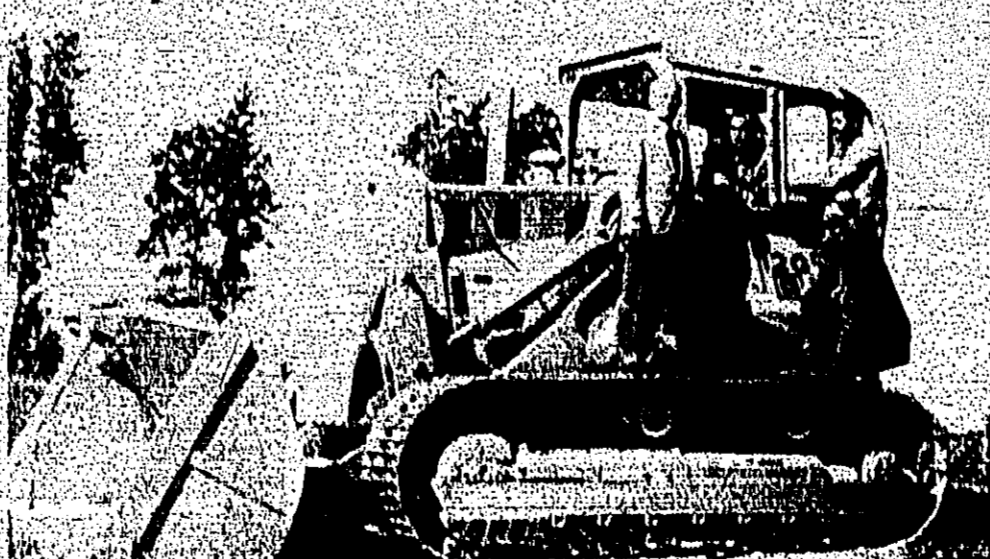
Crawler-loader shown at landfill site—now busy covering solid waste.
