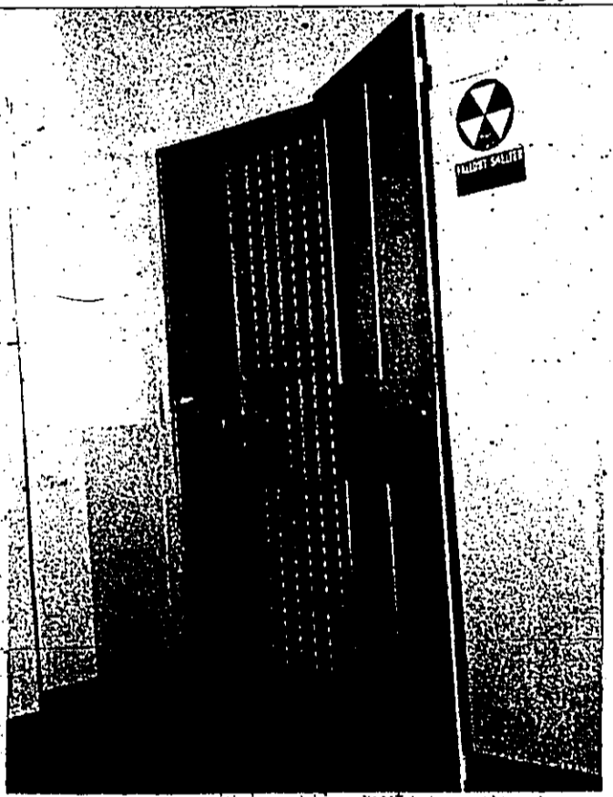
The jail doorway opening into a public corridor is one of the complaints the state inspectors had against the existing facilities.
