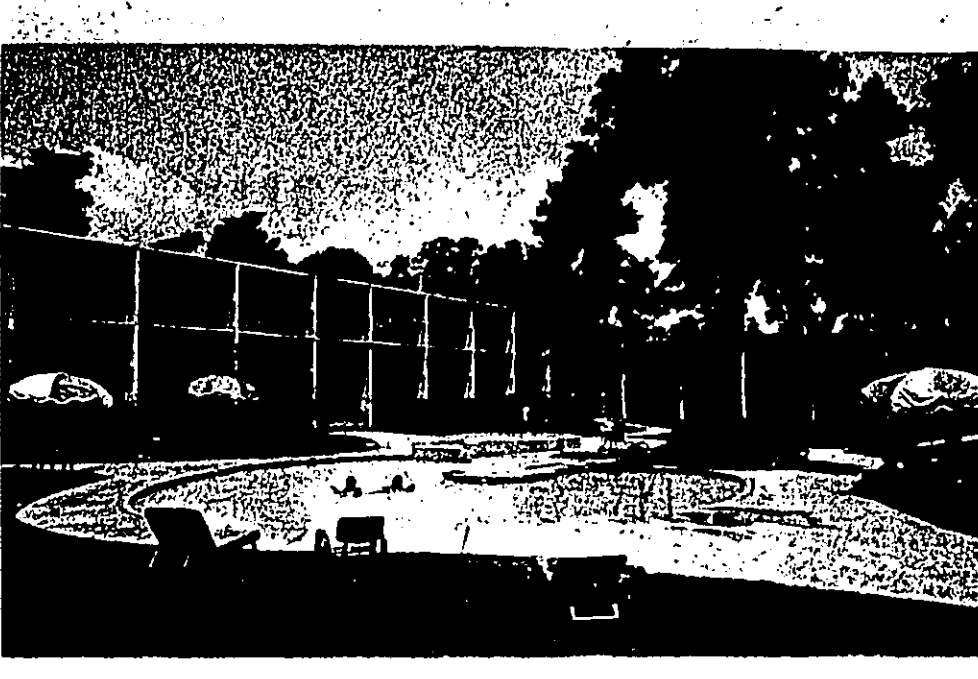
WOULD YOU BELIEVE—it's in Downtown Woodville? It is—and it's a part of the Woodville Inn complex which consists of 72 modern rooms, restaurant including banquet facilities for 400, a gift shop and other modern innovations seldom found downtown in a small city. We should be proud of this unique motor-hotel.
