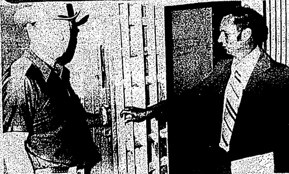
State Jail Commission Officer Bob Derring points out to County Sheriff Lewis Craven, one of the many safety corrections needed in the jail facility. Here, door stops are needed to prevent the heavy iron doors from crushing the jailors fingers should a prisoner suddenly kick the door open when the prisoner is being moved from the cell for some reason.
