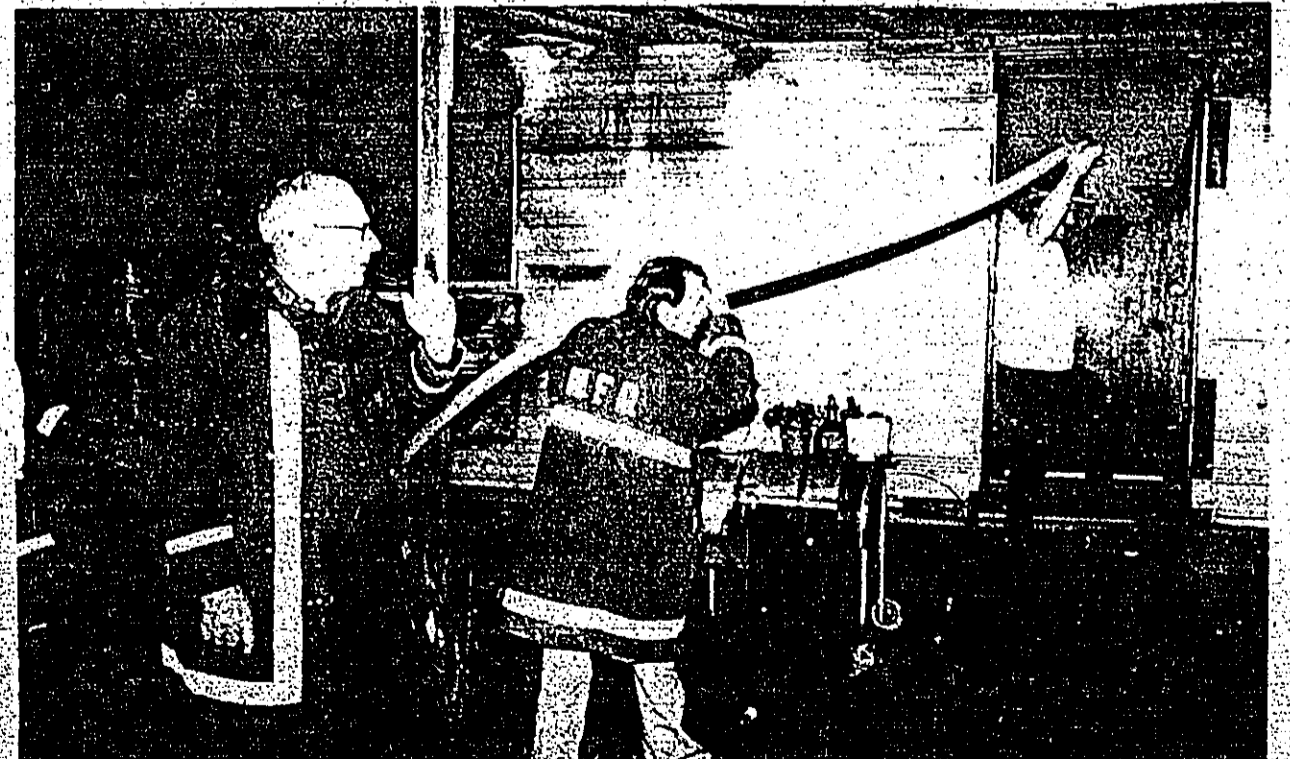
'HOT SPOT' —A mobile home fire on Railroad Street in Southeast Woodville summoned the Woodville Volunteer Fire Department at about 10:30 p.m. Monday. According to Fire Marshall Alva Cook, approximately 1,500 gallons of water were used on the blaze which was considered a "total" loss to Edward (Tex) Lewis, owner of the home. Cause of the fire according to Cook was listed as "unknown." Firemen surmise that the blaze originated in the bedroom which was considered the "Hot Spot" when the firemen arrived.
