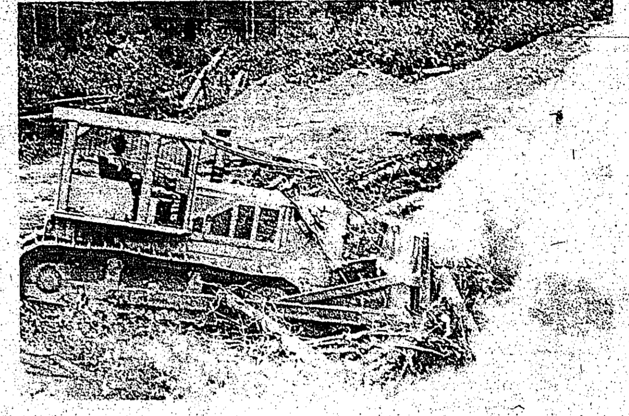
RISKY JOB -Bulldozers push the material into the fire which is being "speed burned" for rapid decomposition. The Texas Forestry Service expressed concern Friday that the experiment will show that the Air Curtain Destructor method of burning material will prove too expensive for operation in East Texas. The method also still produces some harmful gasses from the fire.
