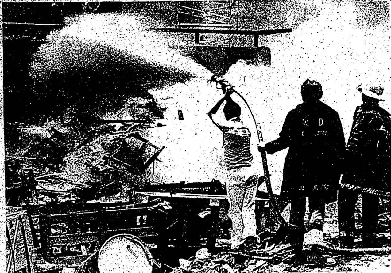
KELLER BLAZE TAPPED OUT —Threatening the main part of the Keller Building, the rubbish fire shown above, got out of hand around noon on Saturday and required the attention of the Woodville Volunteer Fire Department. Quick response by the volunteers had the fire watered down and the plant out of danger in a short time.
