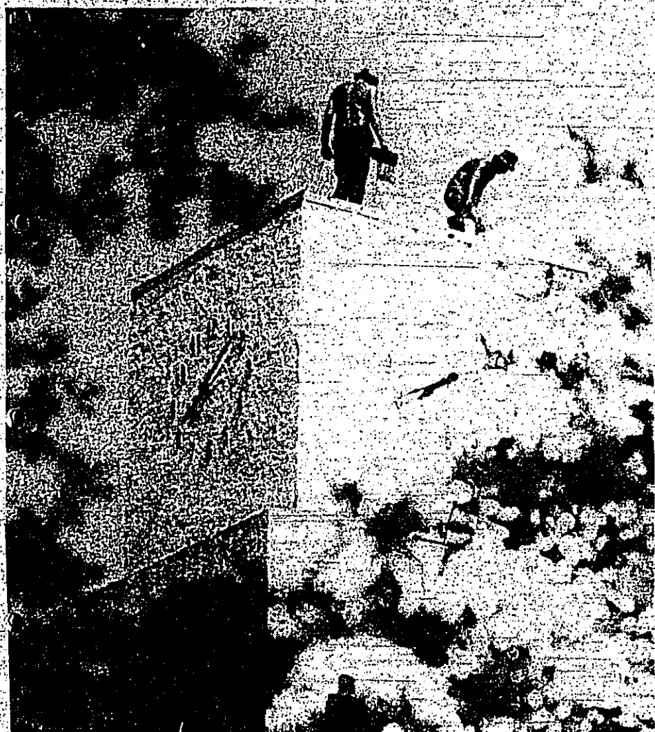
FINISHING TOUCHES —Workmen put the finishing touches on the Tyler County Courthouse roof Monday completing a lengthy rehabilitation project which costs nearly $25,000. The project called for a major portion of the old roof system to be torn out and replaced with new roofing material.
