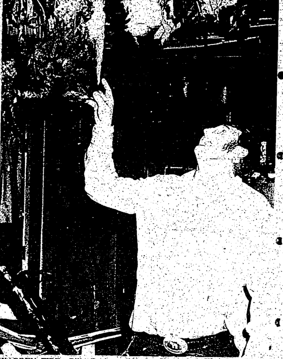
WARREN FIRE —Billy Burks, volunteer fireman at Warren, surveys damage to interior of a house that caught fire Friday south of Warren. Burks said the extensive damage was done to the R. A. Smith residence, south of the overpass on Highway 69. Other Warren firemen responding to the call were Roy Redman and Harold Davis. The Woodville Fire Department also assisted with the blaze and Burks said he would like to thank the Woodville firemen for their cooperation.
