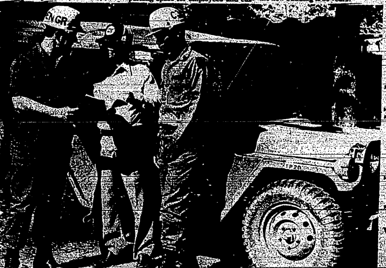
SHELTERED WORKSHOP REMODELING CREW -- Company "C" Soldiers from the 34th Engineer Battalion Ft. Polk, Louisiana, were on site Monday with a group of 26 men and a convoy of heavy duty earth movers to help the Tyler County Mental and Physical Handicap Association open, officially on Monday, June 2. Shown in photo above are Job Superintendent Staff Sergeant Thomas Davis (left), TCM&PHA Director Paul Walker (center) and Electrician Specialist Sergeant Leroy Wells. Officer in charge of the civilian affairs project for Fort Polk is Lieutenant Walter Pierce.
