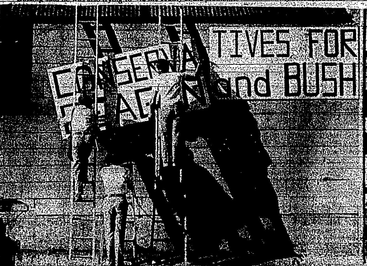
THE WORD'S OUT - Conservatives For Reagan and Bush were out hanging a sign on their headquarters located at the intersection of Hwy. 69 and 190. Shown installing the sign on Monday are Dr. Brian Babin, Jack Whitmire and Jimmy Allison.
