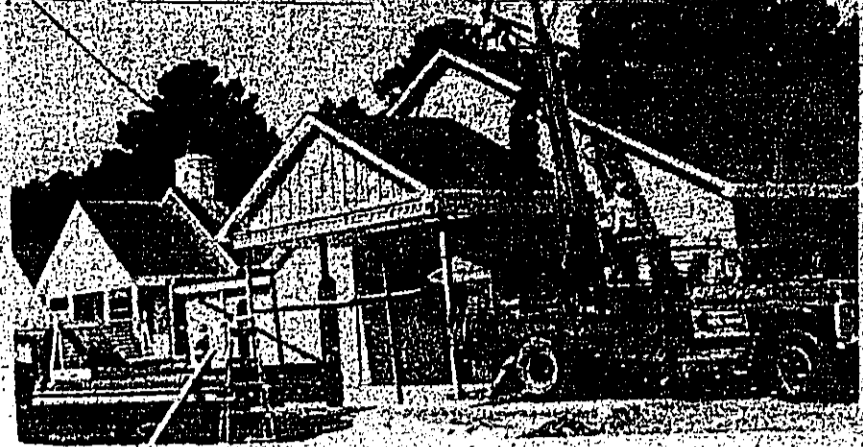
Steeple Placement...Workers lift the steeple into place atop newly constructed First Baptist Church sanctuary facilities in Colmesneil. The new church will formally open its doors this Sunday.
