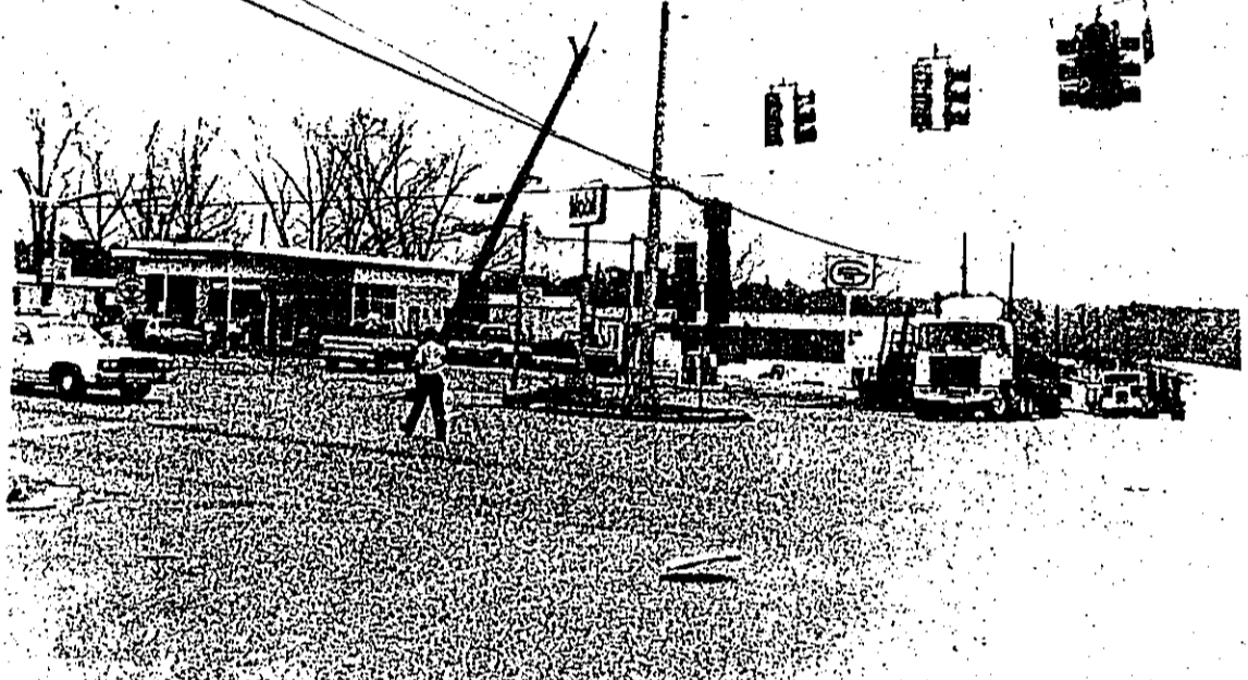
LIGHTS OUT--Workmen from Gulf States Utilities, Southwestern Bell Telephone and American Cablevision worked feverishly Monday night after a log truck failed to negotiate a turn northward from Highway 190 impaling the lower portion of a high capacity telephone and electrical pole located on the Hensarling Mobil Gas Station corner. The accident makes the timely point of the need to improve the turning accesses on both Hwy 190 and U. S. 69. Service was restored quickly by the utility companies.
