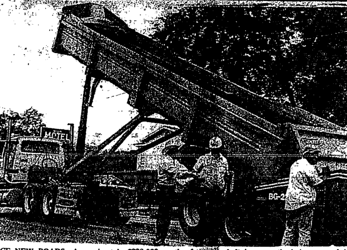
NICE NEW ROADS... Approximately $229,000 worth of asphalt is currently being poured in Woodville on Hwy 69 and 190 by the Highway Department according to Thomas Morgan, Engineering Technician. The work should be completed in a week to ten days depending on weather conditions.
