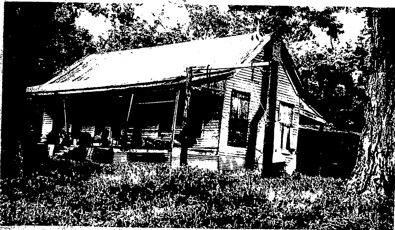
THE RESTORATION OF THE 1835 CAUBLE HOUSE—North of Chester, is just one of the projects facing the Tyler County Heritage Society this coming year as a result of a Grant issued to the Society on behalf of Cauble family members.
