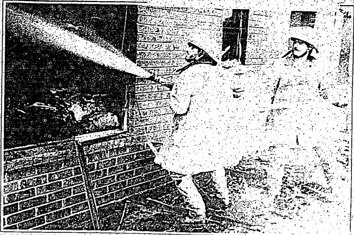
VALIANT EFFORT-- Woodville Volunteer Firemen made a valiant effort Sunday to extinguish the KVLL Radio Station fire. The blaze apparently started in a control room; KVLL's "Sunday" Man, Jerry Wright, of Kirbyville, noticed that something smelled funny, then went to look, noticed smoke, then called for help after barely escaping from the building.
