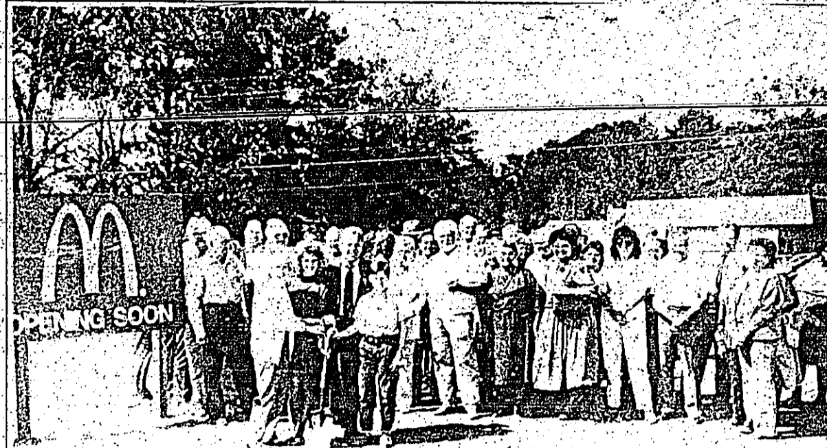
GOLDEN ARCHES IN WOODVILLE- Chamber officers and local dignitaries watched as the first shovel of soil was turned by owners, Jack and Suzanne Schwartz at the corner of Hwy 69 and Cobb Mill Road.
