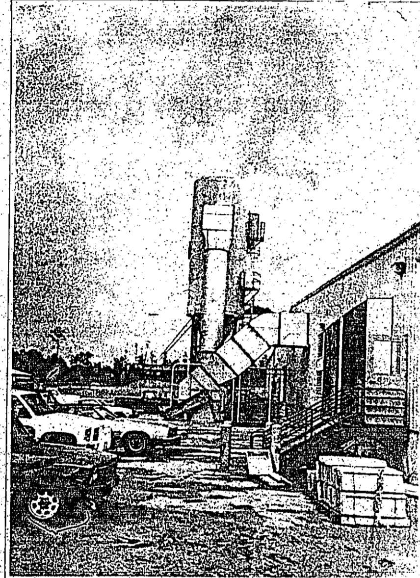
A shot of the shipping and receiving area of the woodworking plant on the Gib Lewis Shrot Unit site.
