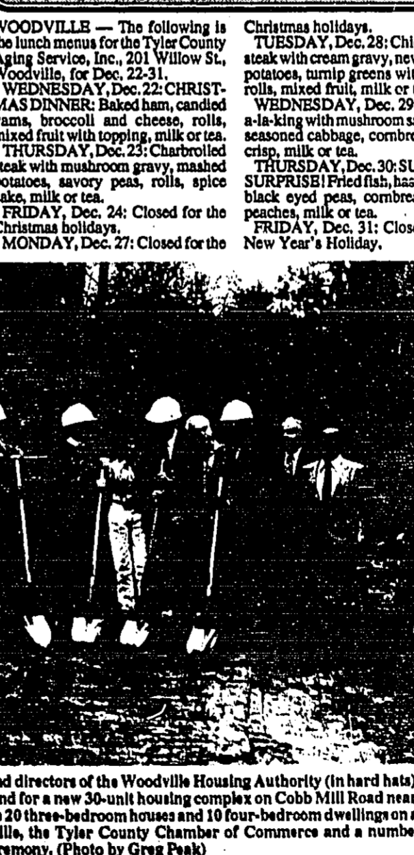
GOLD SHOVEL TIME — Officials and directors of the Woodville Housing Authority (in hard hats) took gold shovels in hand Monday to break ground for a new 30-unit housing complex on Cobb Hill Road near Highway 69.
